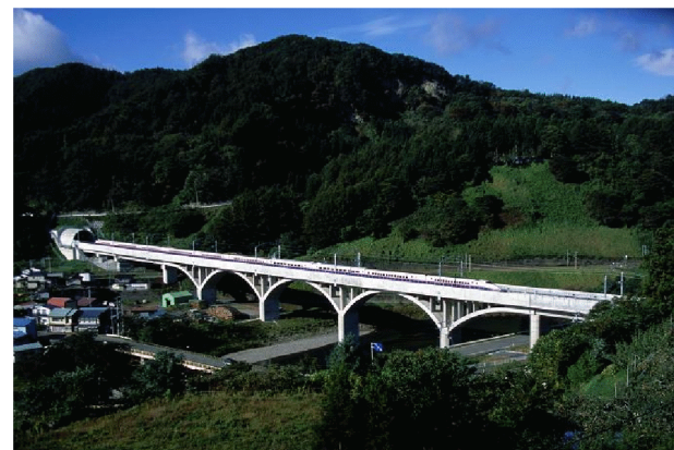
Bridge ( Tohoku Shinkansen )
